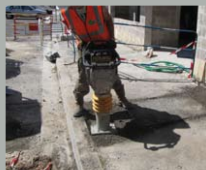
REMBLAYAGE - COMPACTAGE
