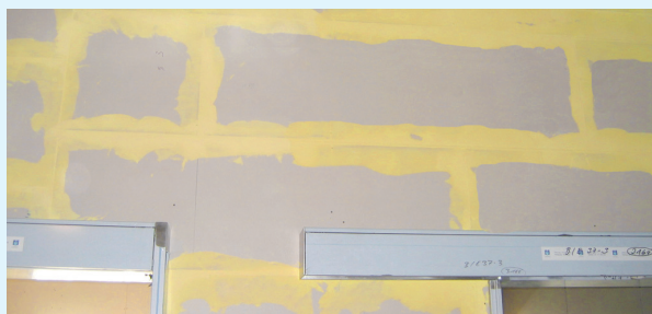
Cloison KM, parements Safeboard + plaque KS de finition
